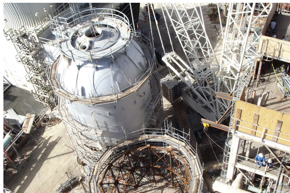
From exchangers to FCCs and cokers, Matrix has been performing full plant turnarounds for more than 25 years.
