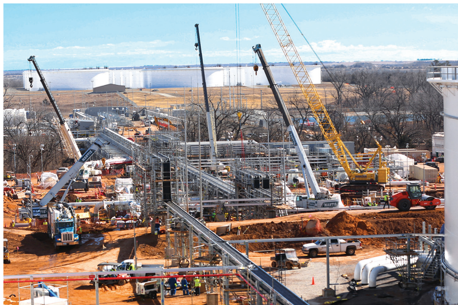
Matrix provides FEED studies, engineering, procurement, construction and fabrication for crude, natural gas, LNG and NGL terminals and also provides specialized engineering as well as procurement and construction at refineries, fertilizer plants and more.
