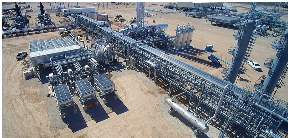
Energy Transfer Partners Red Bluff 200-million-standard-cubic-foot-per-day gas processing facility near Orla, Texas, where Matrix PDM performed balance of plant engineering, design, procurement and project management.
