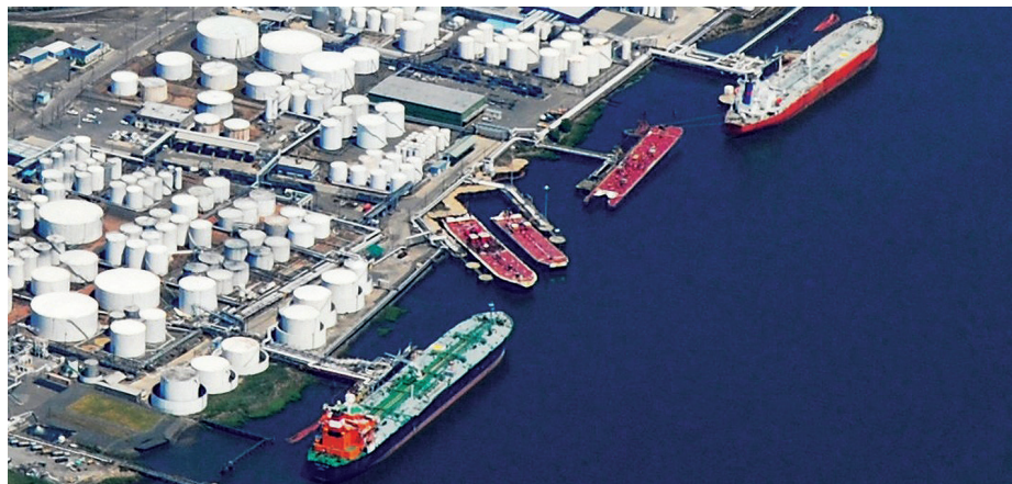
Kinder Morgan flagship northeast terminal in New York Harbor, where Matrix PDM provided engineering and project management for upgrades and expansion of barge and ship loading and unloading facilities.
