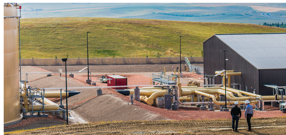
Matrix Service Inc. General Manager of EPC James Prette, left, and Energy Transfer Partners Vice President of Liquid Engineering Chuck Frey on-site at the Dakota Access Pipeline Johnson's Corner terminal.
