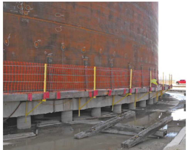
Figure 4. Elevated pile cap foundation.
