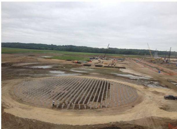
Figure 5. Formwork sand installation for elevated pile cap.
