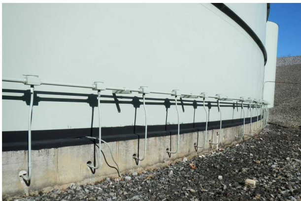
Figure 7. Foundation heating system.
