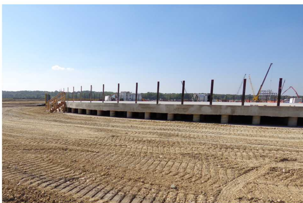
Figure 6. Elevated pile cap after formwork sand removal.
