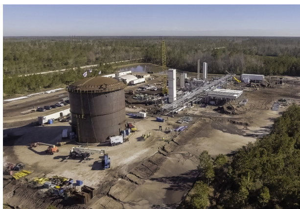
Figure 2. Eagle LNG's Maxville LNG facility near Jacksonville will be used to liquefy and store LNG used for ship bunkering.
