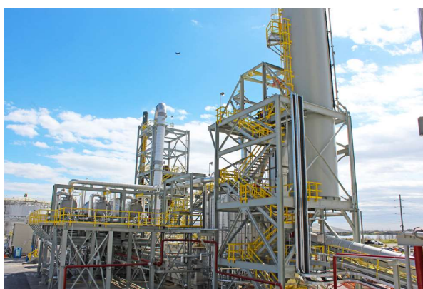
Figure 3. A 1 million tpy sulfur remelter with lime silo, external heat exchangers and a scrubber.
