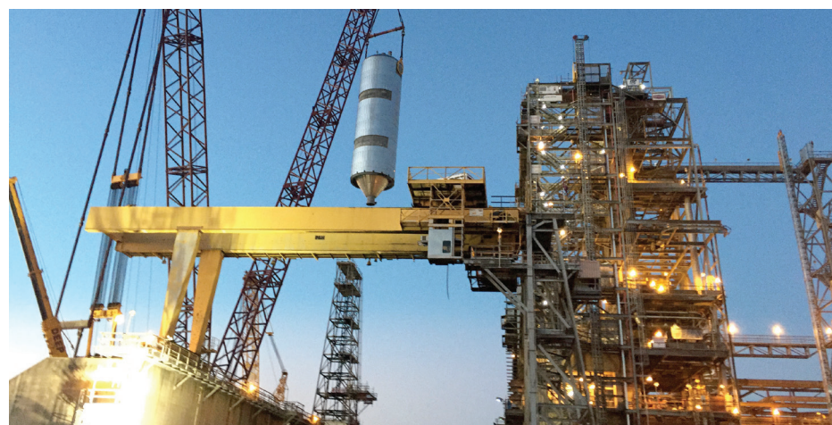
Maya II's coker drums represented part of over 6 million pounds safely lifted during a 12-day period of the turnaround.
